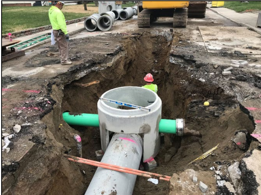
The City of Noblesville has announced its Long Term Control Plan Phase 5 work wrapped up on 16th Street on Wednesday. The work included installing a conflict structure manhole. According to city officials, there are various utilities that conflict in this area. Crews have begun saw cutting the asphalt on 14th Street and will start construction on Thursday to install the new storm pipe from Conner Street to Maple Avenue. City officials said that because of the narrow complexity of 14th Street, it may need to be closed through the weekend and into next week.
