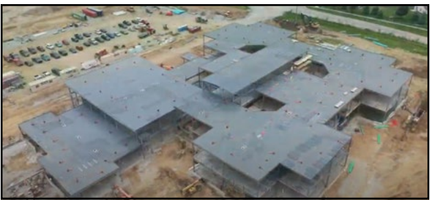
Photo provided Deer Creek Elementary construction as seen in a Hagerman Group drone video.
